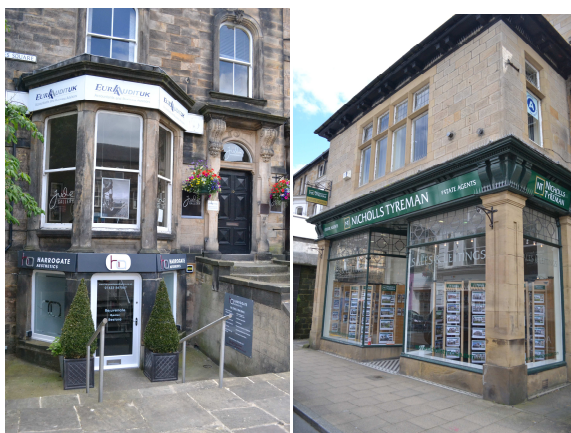
Predominantly with estate agents offices & basement cafe usage
