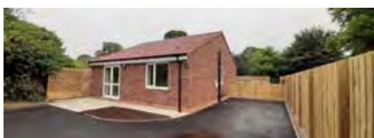
Springfield Drive, Boroughbridge
