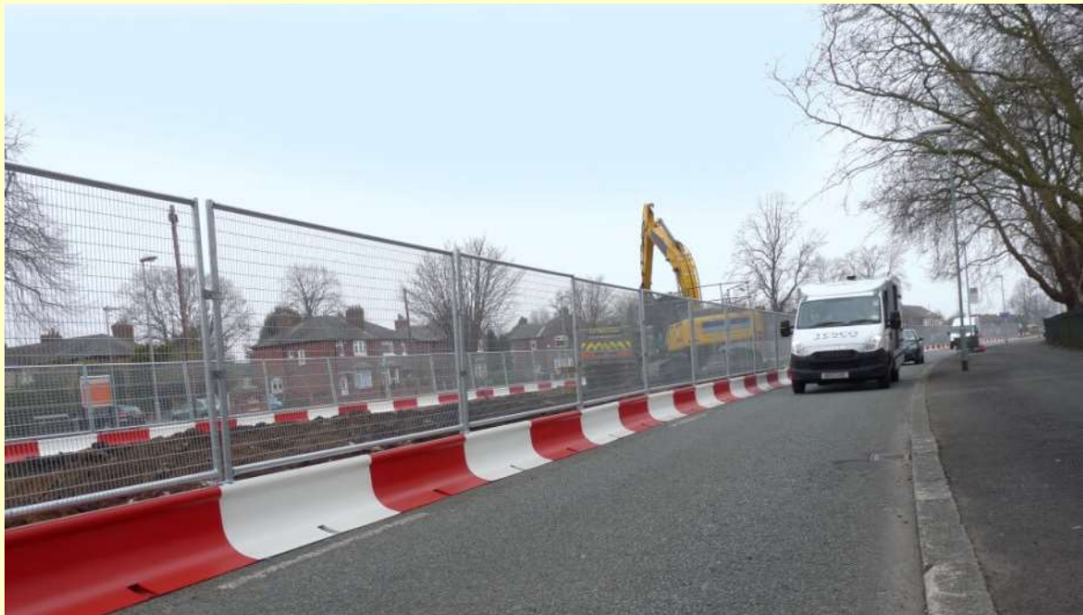
Figure 3-3: Example of a M.A.S.S. Barrier installed
