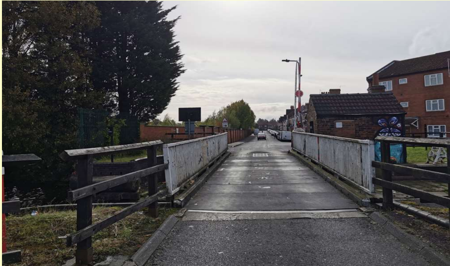
Figure 2-8: Narrow canal bridge at Denison Road
