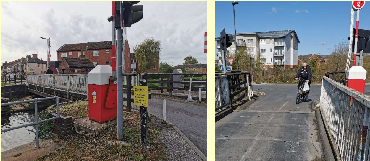
Figure 3-4 – Denison Road Canal Bridge
